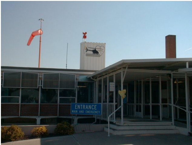
Odessa Memorial Hospital, one of Odessa Office Equipment's commercial customers. The wireless equipment and router (to interface to the hospital's existing network) is located in the elevator shaft. The square, flat panel antenna is barely visible near the tail of the helicopter logo.
